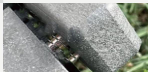
Ordinary stainless steel screws, the color is abruptly exposed, poor stability and easy to rust and rot
